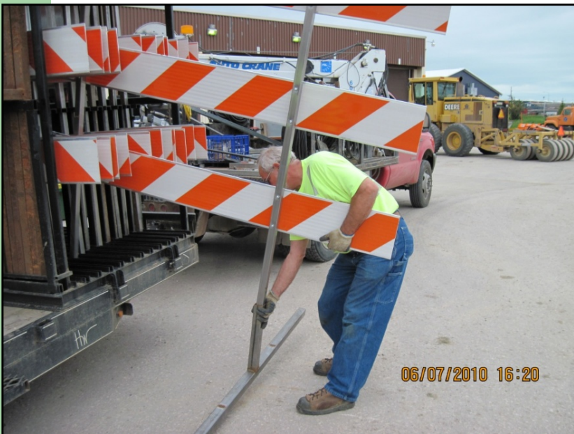
Barricade rack & aids in installing stand
