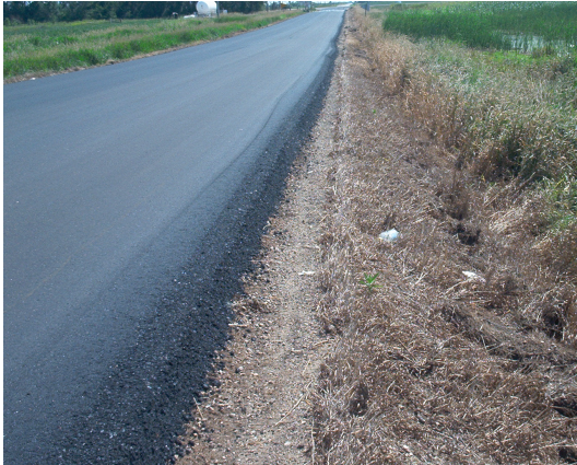
Example of the problem we are trying to avoid – the severe shoulder drop-off when overlay is placed on a narrow roadway.
