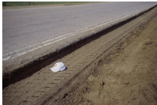
The finished undercut just prior to being filled with new base aggregate.
