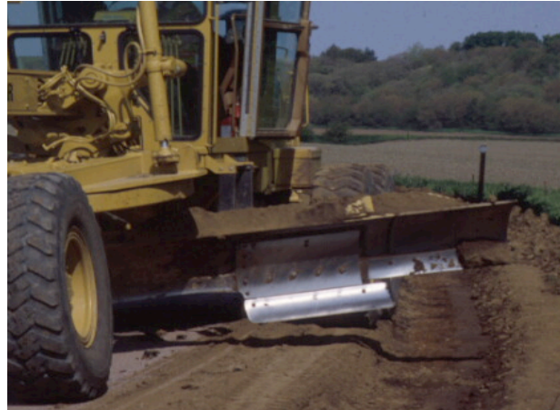
The shop-built device mounted on grader moldboard used to make the undercut.
