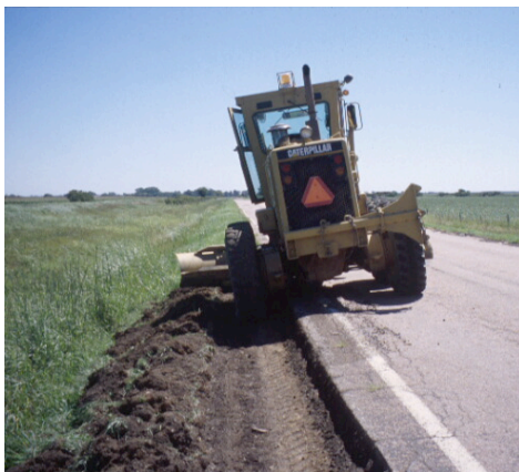
The undercut being made. A grader with a cutting wheel is used prior to this operation to make a straight cut at the edge of the old pavement.
