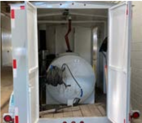
© 2022 Stark County ND, Highway Department
